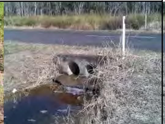
Construction of pipe culverts across the roads within mine lease
