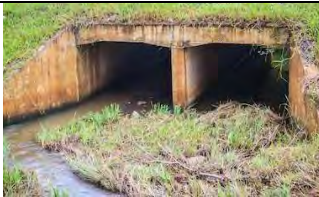
Box Culverts of outside roads
