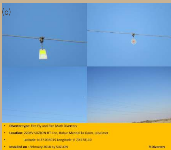
Image 9. Pilot installation of bird diverters on power lines near (a) Khuchdi, (b) Habur- Sanu and (c) Mandal ki gaon villages – priority areas for mitigating power lines for Great Indian Bustard conservation in Jaisalmer, Rajasthan. © Mohib Uddin
