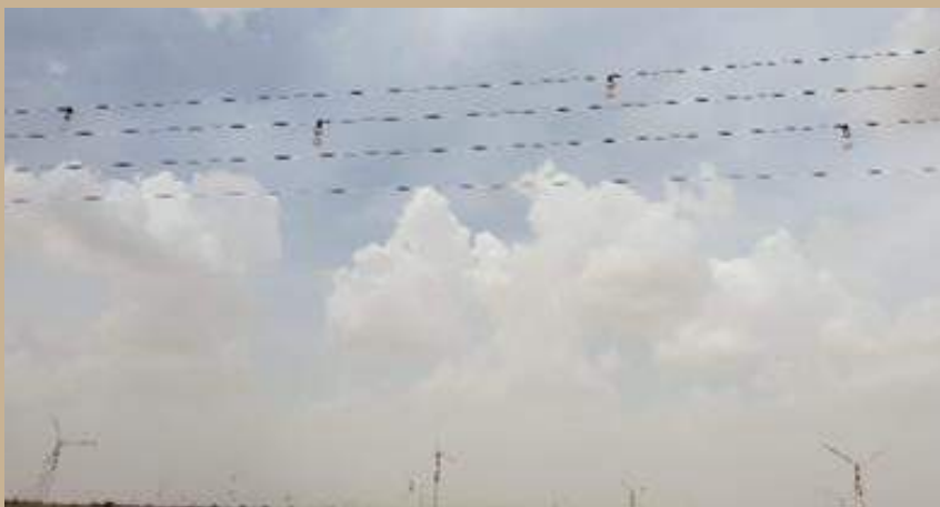
Image 11. Pilot installation of indigenous LED bird diverters according to the design provided by Wildlife Institute of India on power lines in Mokla – priority area for mitigating power lines for Great Indian Bustard conservation in Jaisalmer, Rajasthan. Photo credit: Suzlon and Devendradutta Pandey
