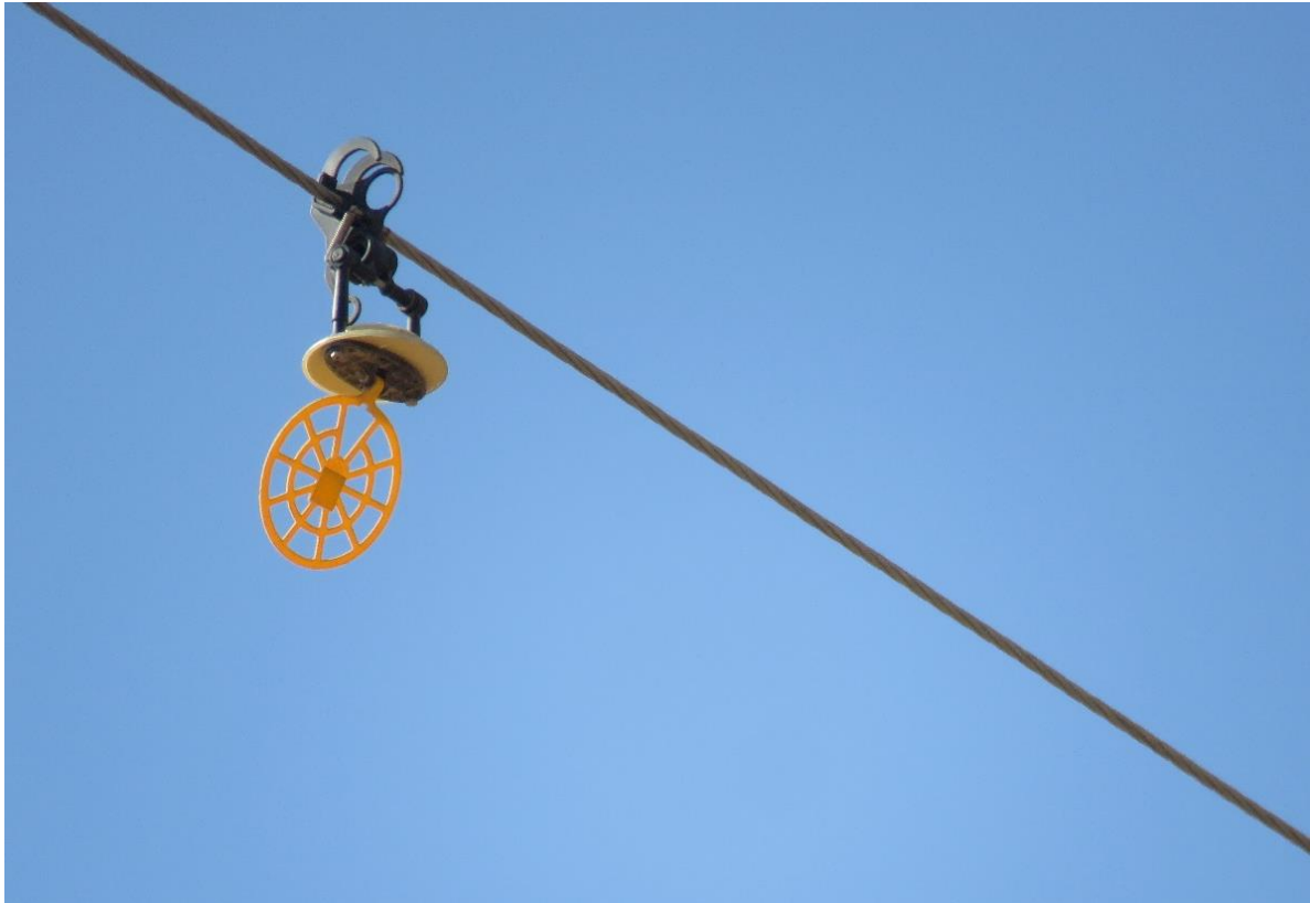
Figure 2. A solar LED equipped bird diverter installed on a powerline in Jaisalmer, Rajasthan.
