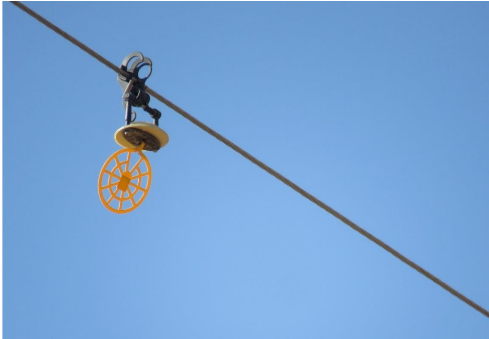
Figure 4. A solar LED equipped bird diverter installed on a power-line in Jaisalmer, Rajasthan.
