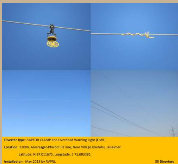
Image 10. Pilot installation of LED bird diverters on power lines near Khetolai village– priority area for mitigating power lines for Great Indian Bustard conservation in Jaisalmer, Rajasthan. © Mohib Uddin and Sourav Supakar
