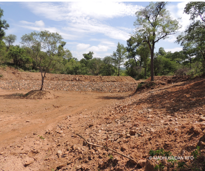
Desilting of water hole
