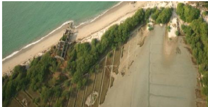
Parallel canal banking tried in Pamban
